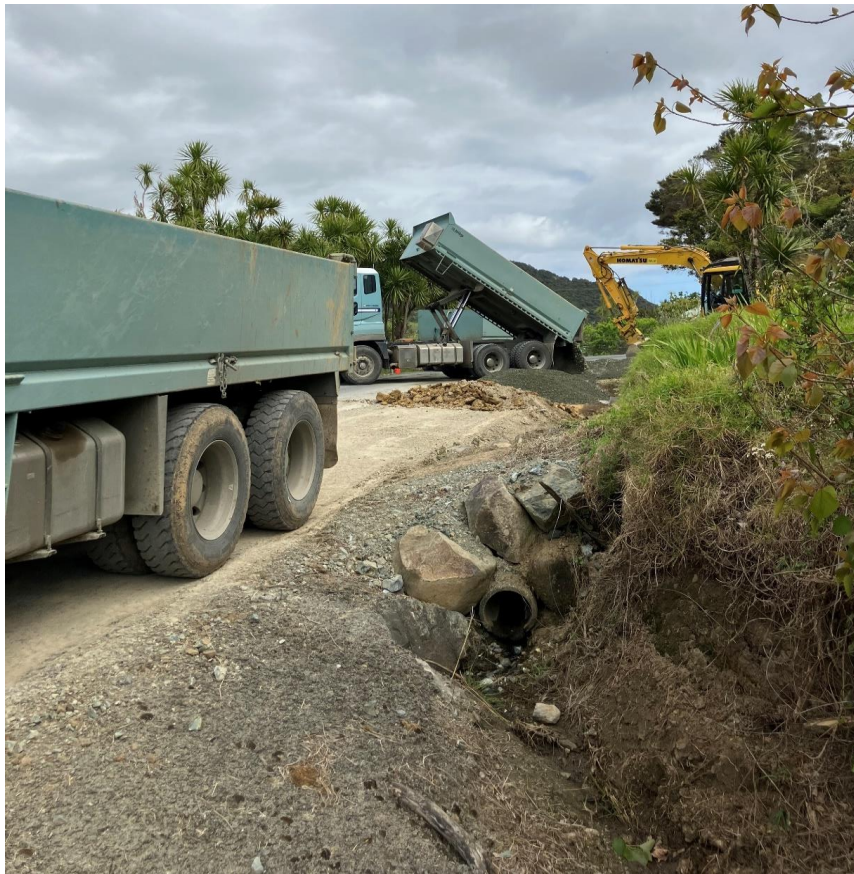
Figure 1: Pavement repair in progress Tauranga Bay Rd, in preparation for an upcoming reseal
