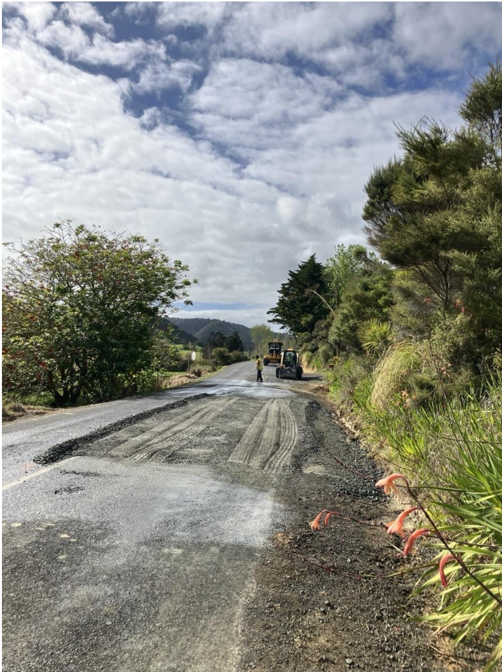
Pre-reseal pavement repairs in progress Tauranga Bay Rd
