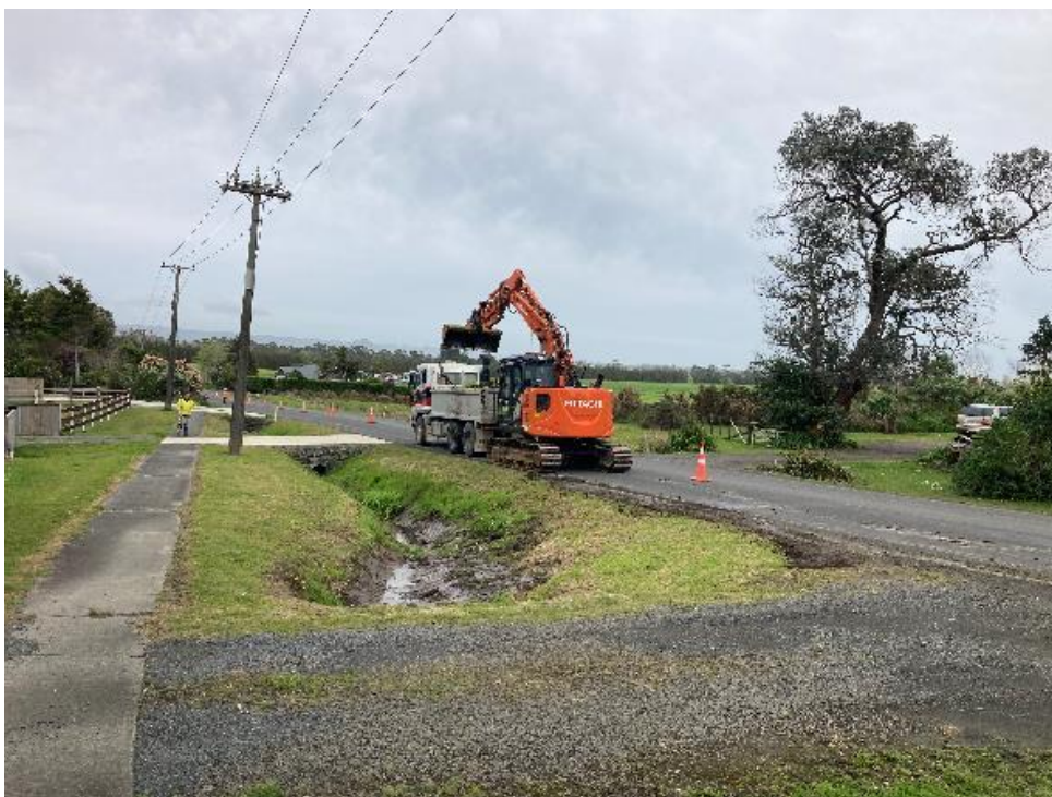
Figure 1: Drainage improvements on Kaitaia Awaroa Rd in preparation for an upcoming reseal
