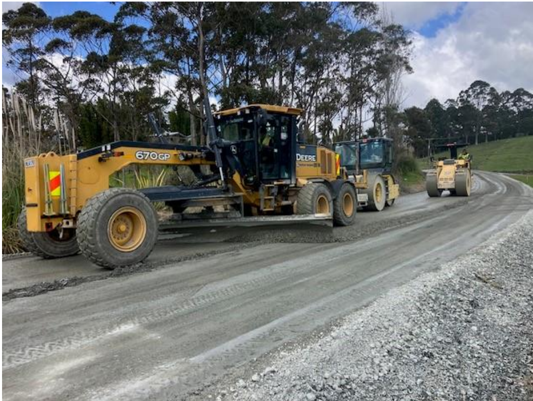
Pavement seal preparation in action on the Ruaroa Road Seal Extension. This is our first renewal project completed for the season, with 900m of new seal completed.
