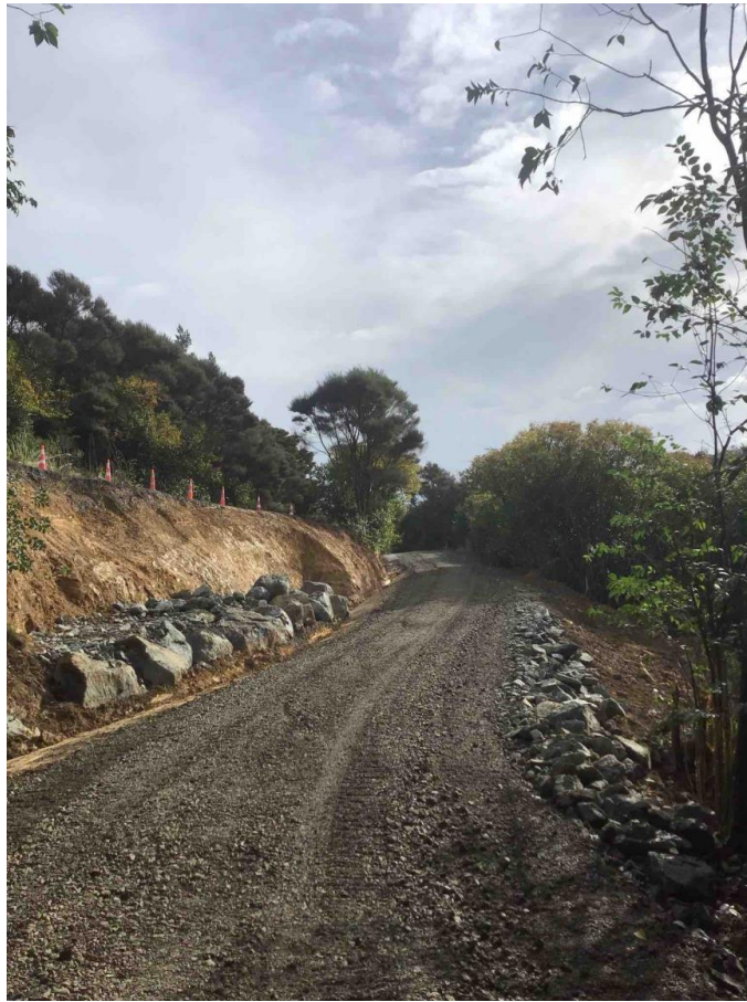
Fryer Rd Rock Wall in progress
