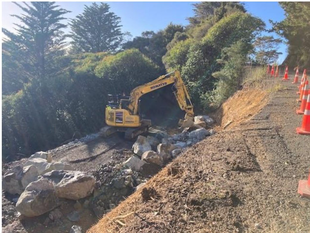
Figure 1: Slip Repair in progress – Fryer Rd, Kaitaia
