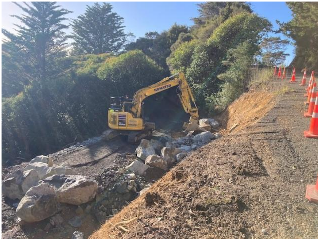
Figure 1: Slip Repair in progress – Fryer Rd, Kaitaia
