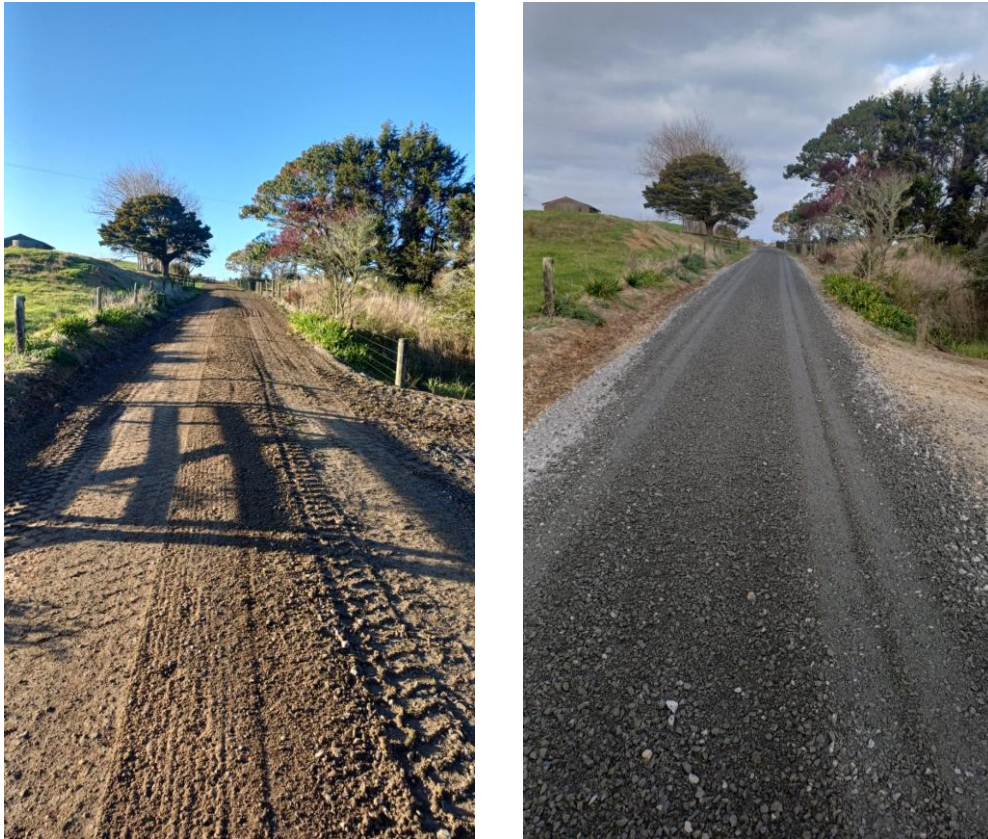
Russek Road before / after
