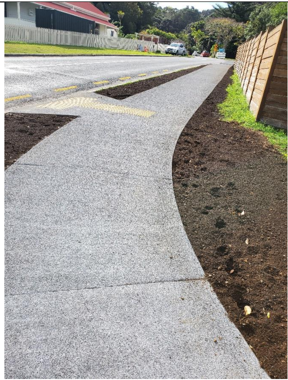
7-23-187 Queen Street New Footpath – Complete
