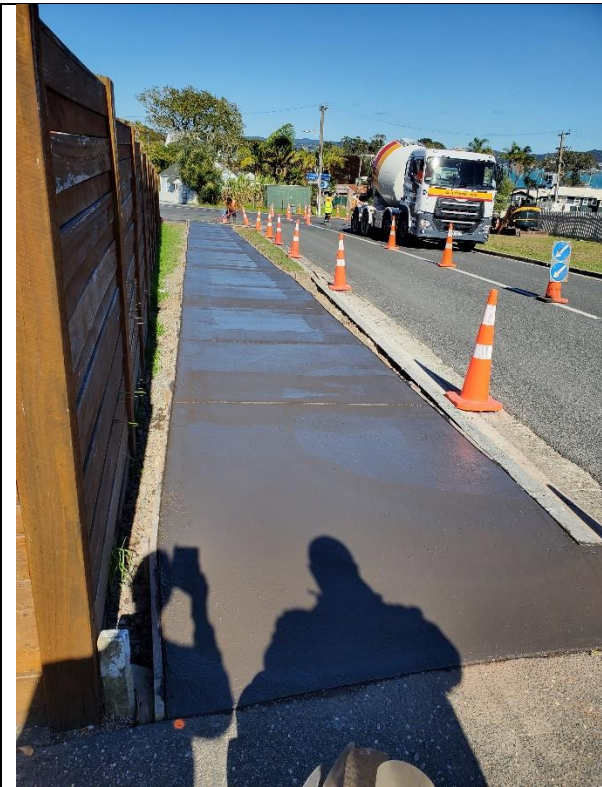
7-23-187 Queen Street New Footpath – Concrete down
