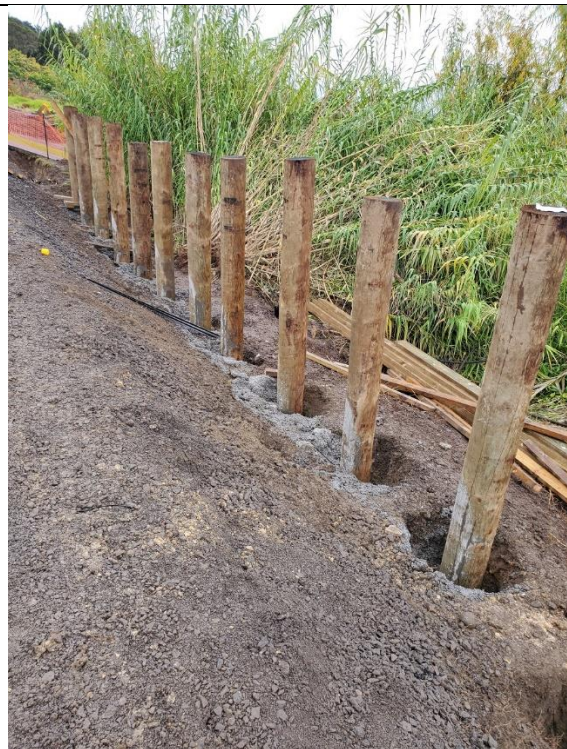
7-23-188 Parnell Street, Rawene – Second retaining wall started
