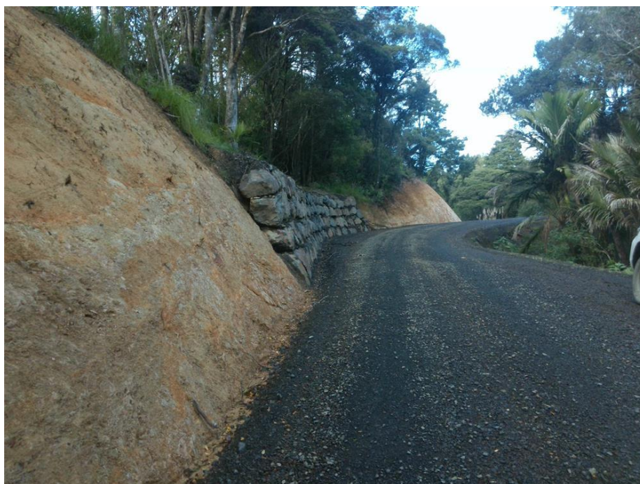
Over slip repair completed on Waiotehue Road by Far North Roding crew.
