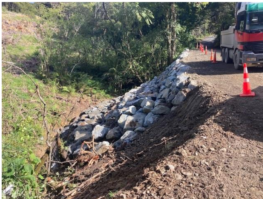
Slip repair completed on Diggers Valley Road by Mike Harrison's Digger Solutions and crew.
