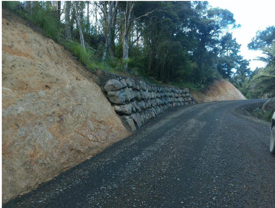
Over slip repair completed on Waiotehue Road by Far North Roding crew.
