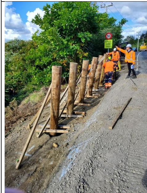
7-23-188 School to Honey Street section, Rawene. Retaining wall post for new footpath, inspection.
