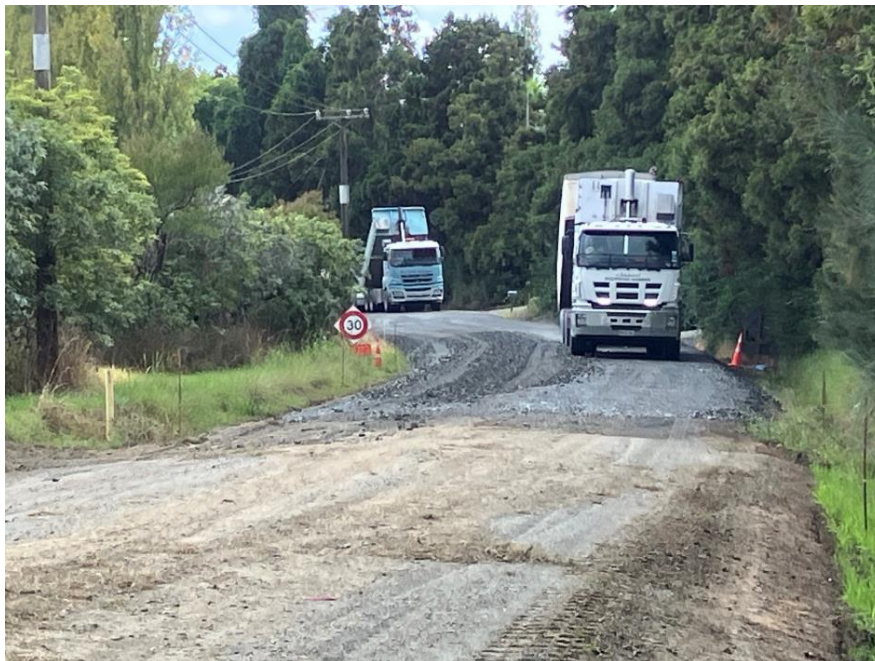
Overlay in progress Ruaroa Rd Seal Extension
