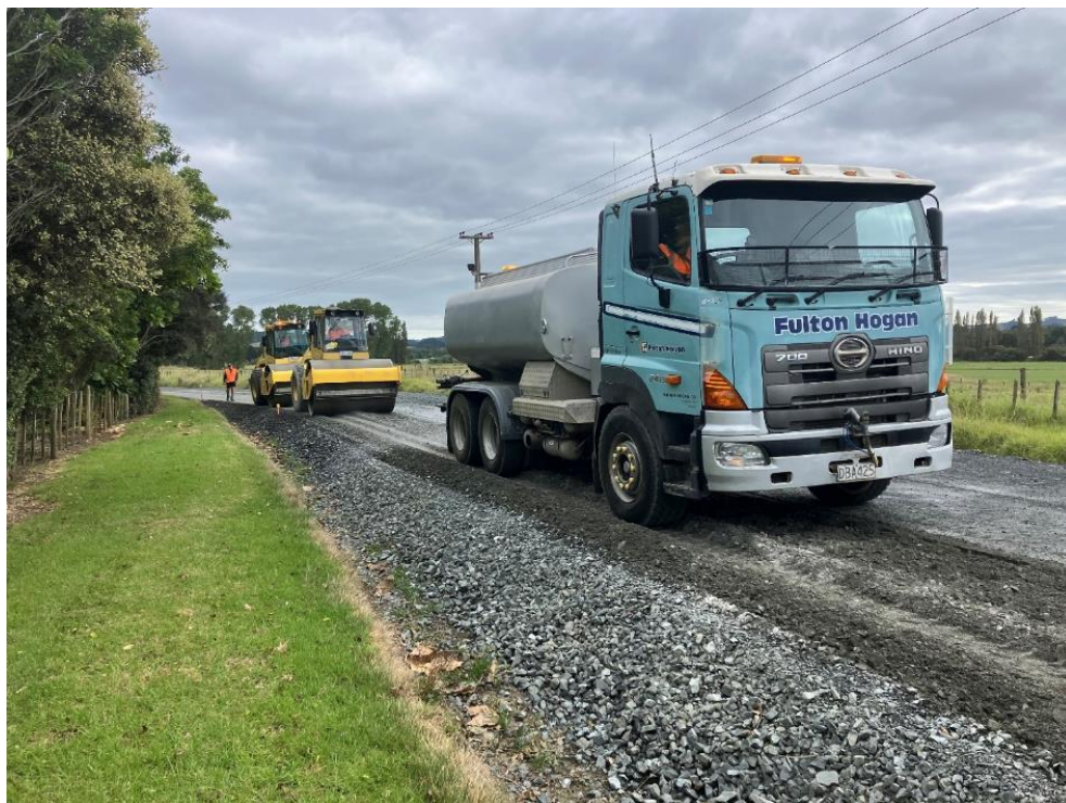
Stabilisation in progress Ruaroa Seal Extension
