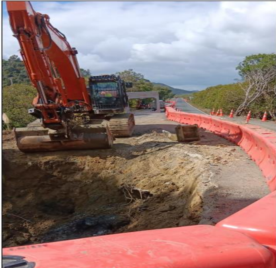
Figure 4 Whangaroa culvert replacement with portable traffic signals reducing the road down to one lane
