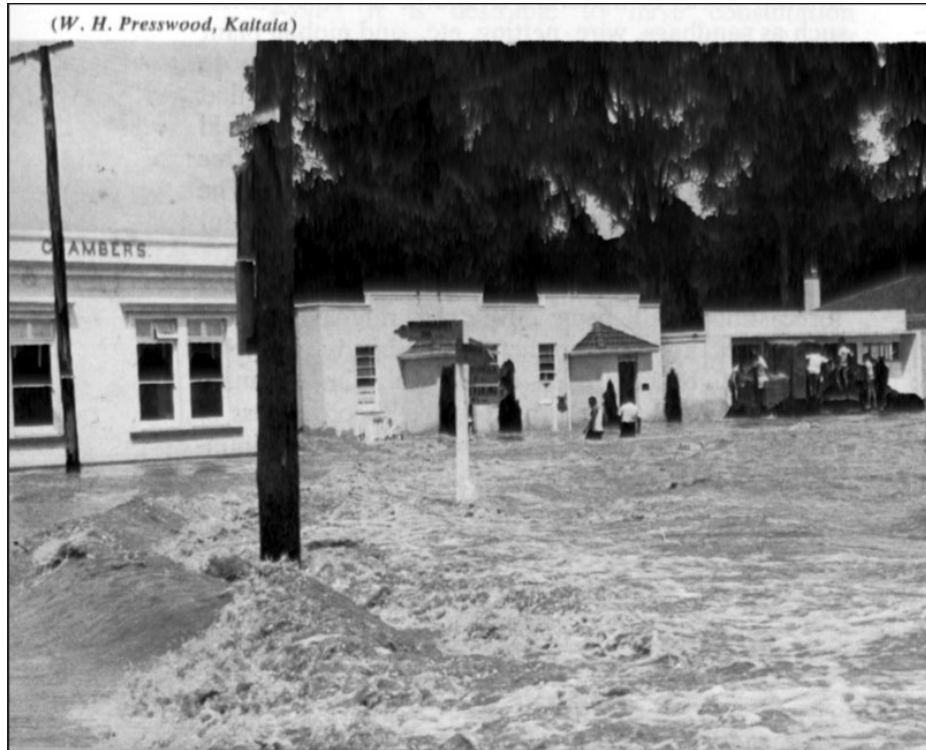
1958 Flood – Commerce Street, Kaitaia (various)
