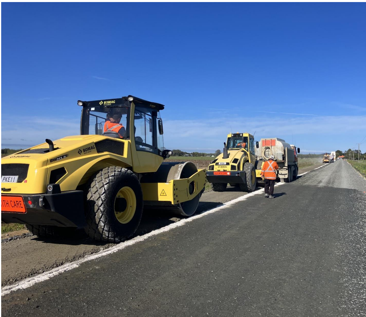
Stabilisation of the Gill Road Pavement Rehabilitation
