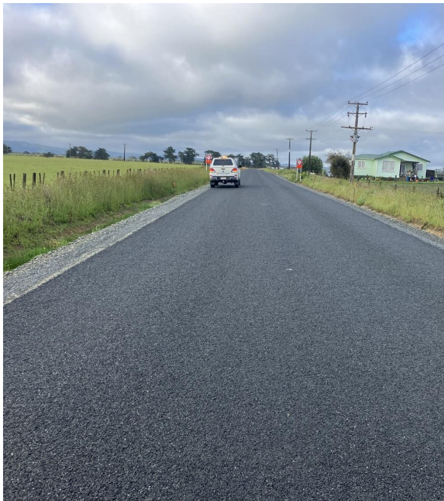
Gill Rd Pavement Rehabilitation Seal
