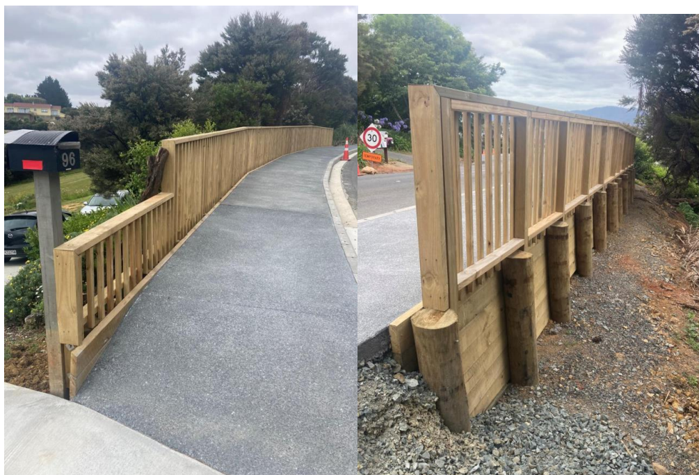
Cable Bay Block Rd New Retaining Wall and Footpath
