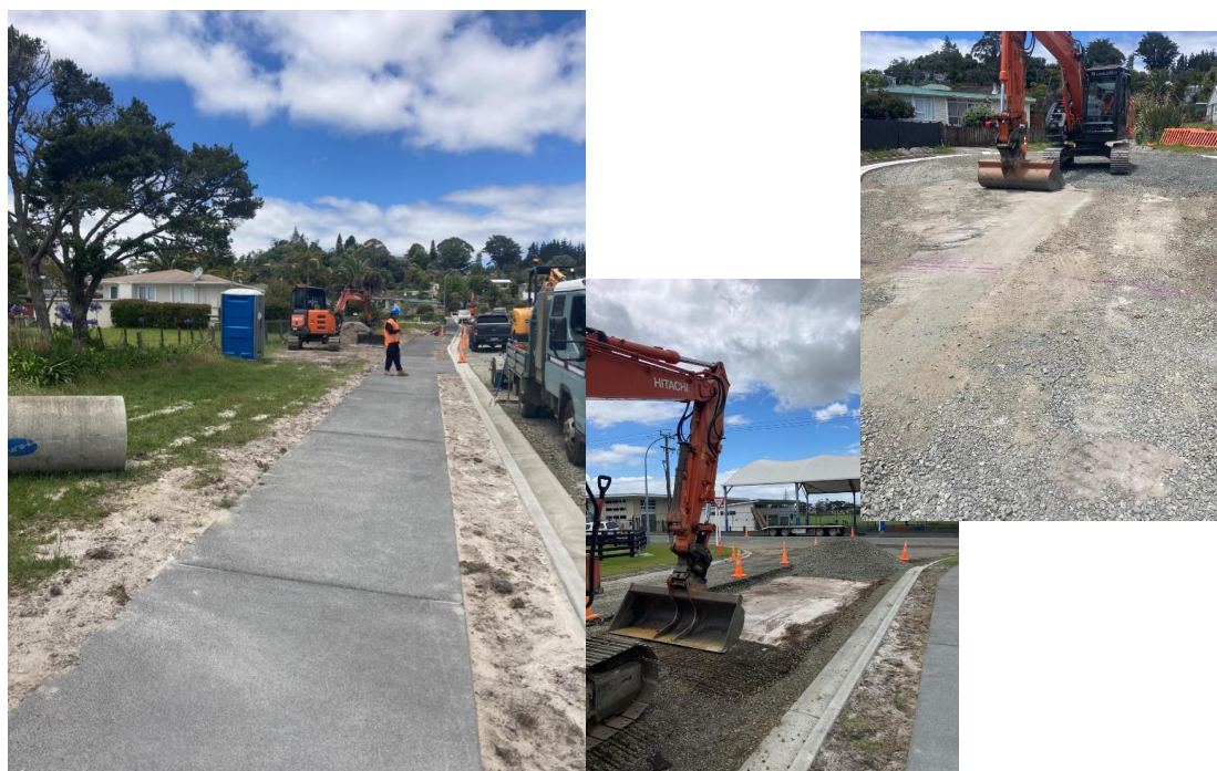
Sommerville Ave Kerb and Channel, Footpath and Pavement Construction
