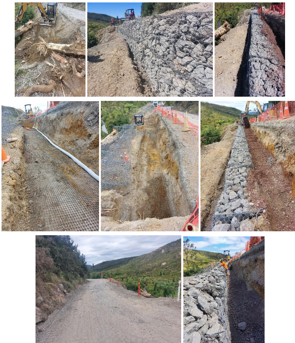
Pipiwai Rd Under slip repair
