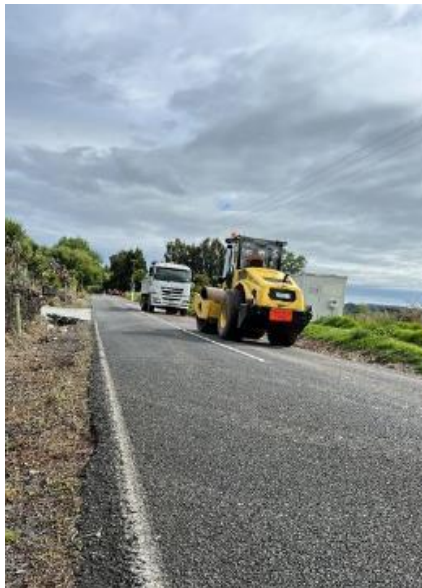
Preseal Repairs Keri inlet Rd / Waiomio Rd
