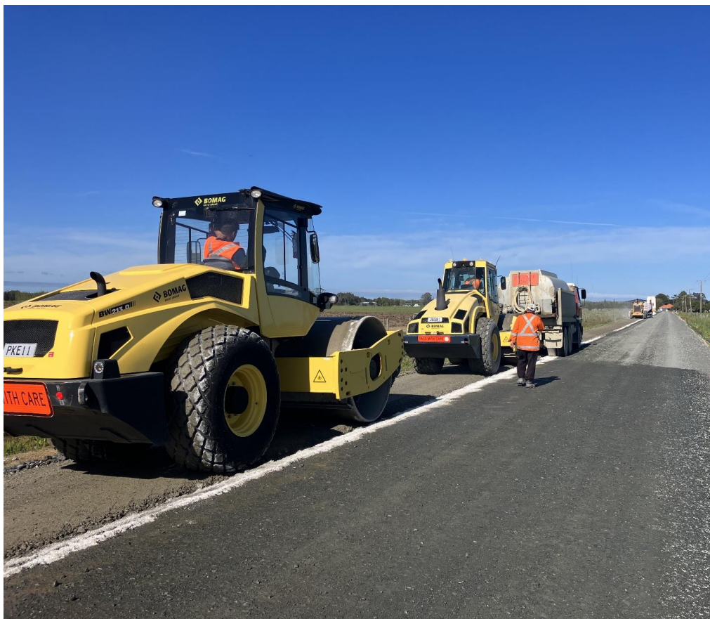
Stabilisation of the Gill Road Pavement Rehabilitation
