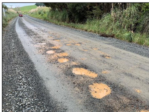
Figure 8.4.1 – Multiple potholes in southern end of road
