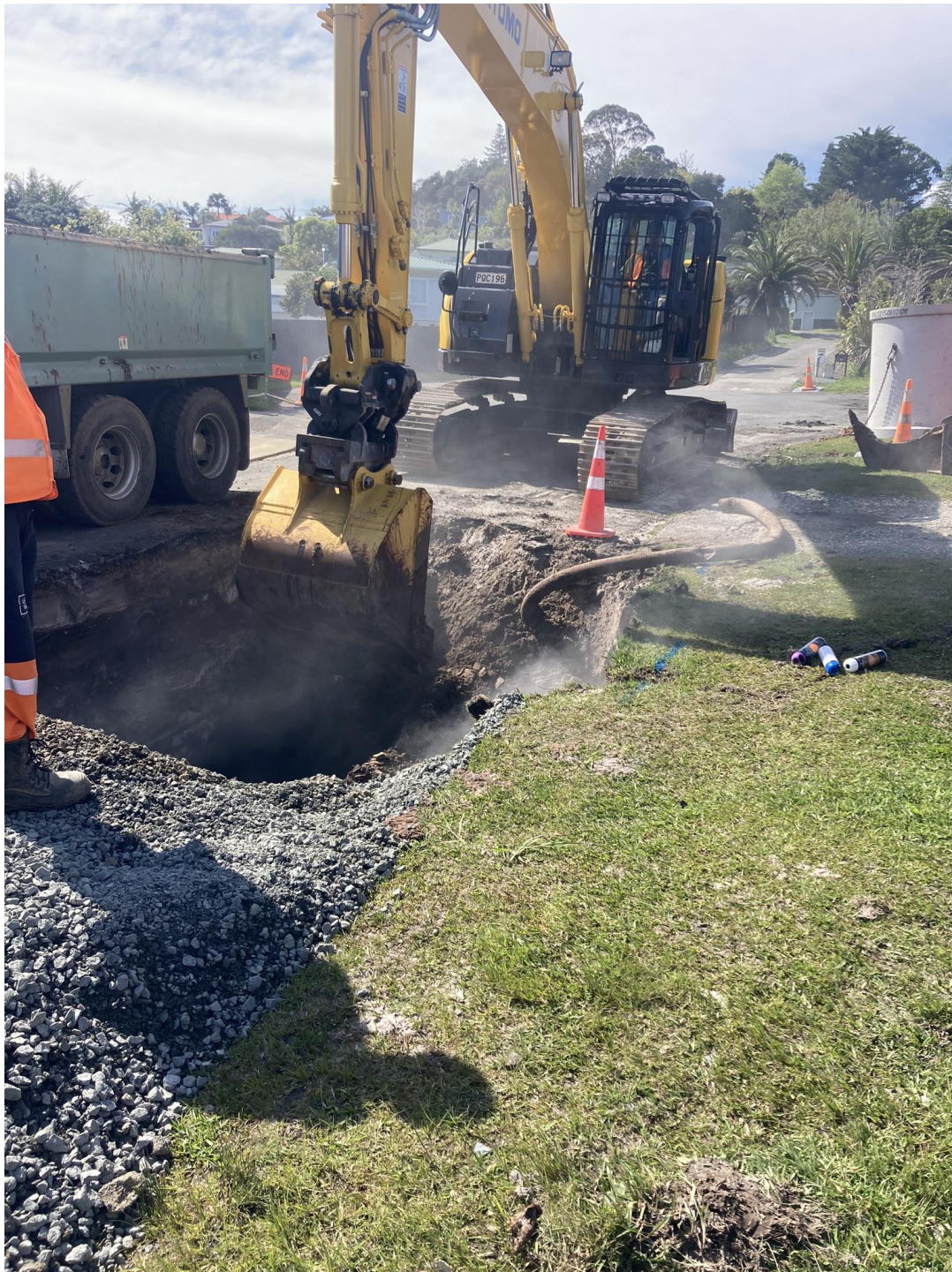
Sommerville Ave SW Upgrade Installation
