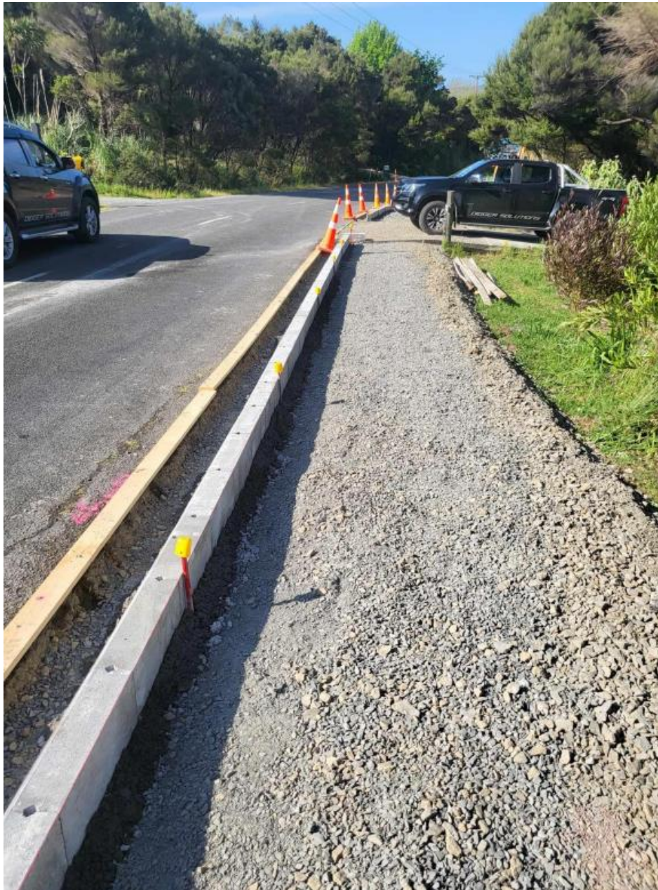
Cable Bay Block Road New Footpath Prep
