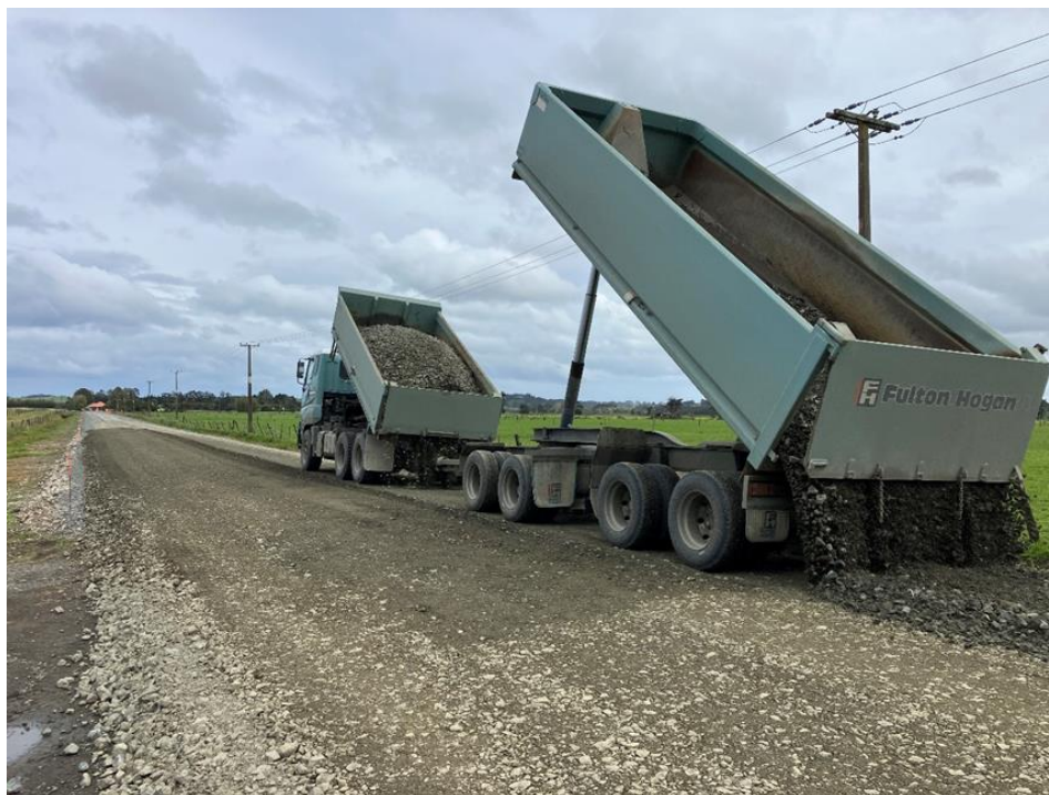
Gill Rd Pavement Rehabilitation Overlay
