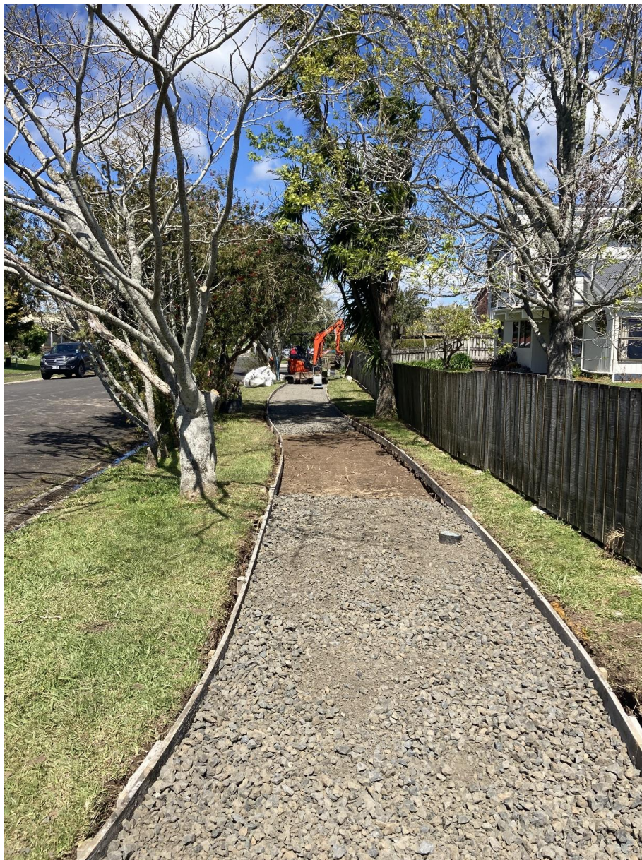
Contract 7/18/100 FNDC North Road Maintenance & Renewals
