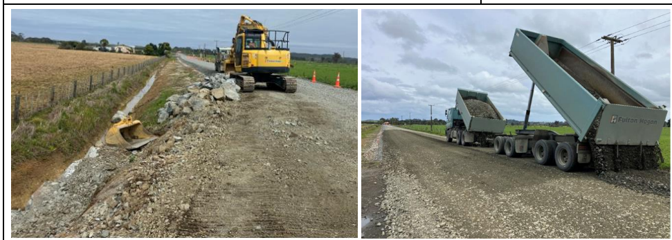
Gill Road Rehabilitation Awanui Rockwalling to support shoulders (left) and overlaying of pavement (right)
