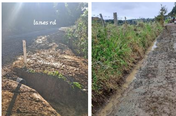
Lanes Rd Culvert Renewal / Omanaia Rd Water Tabling
