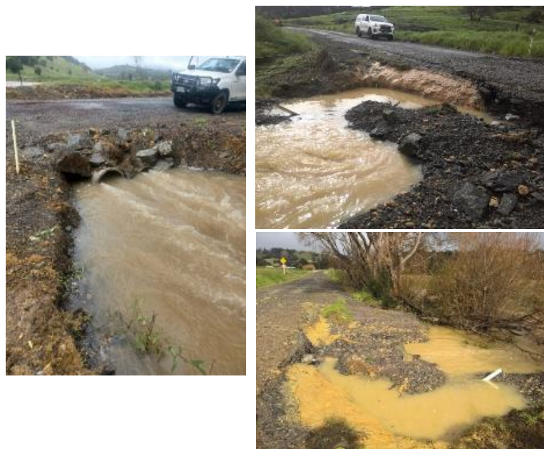
Before/After Tipene Rd Culvert Renewal
