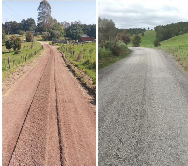
Pinehill Rd / Inksters Rd Maintenance Metal
