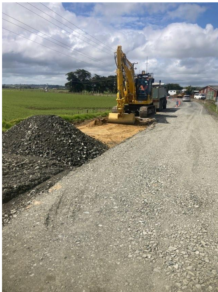
Gills Road Pavement Rehab Pavement Undercuts
