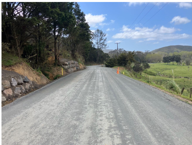
Pawarenga Rd Seal Extension Prepped for Seal
