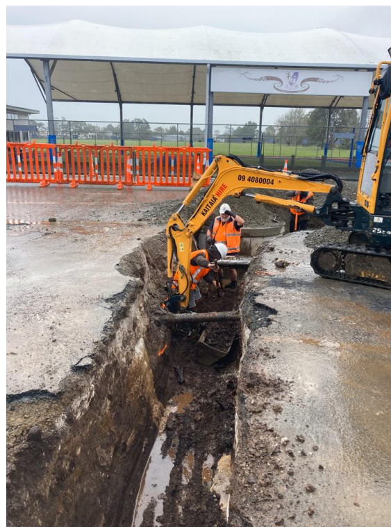
Sommerville Ave SW Upgrade Pipe Installation
