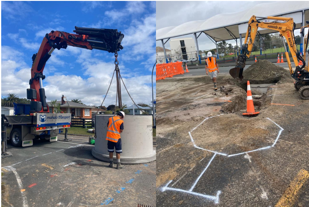
Sommerville Ave SW Upgrade Manhole Delivery and Installation
