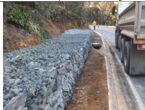
Gabion Wall (Cove Rd RP16,000)
