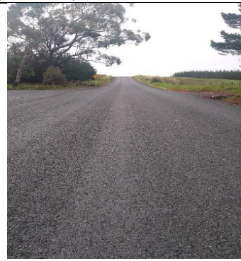
2 nd coat reseals on Pouto seal extension
