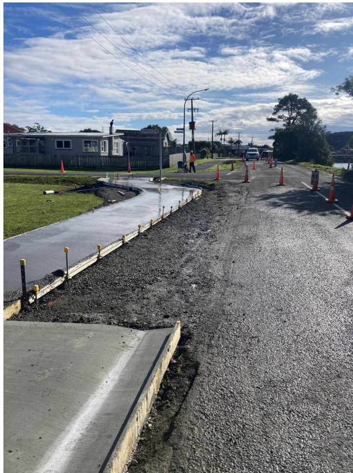
Oruru Road New Footpath Construction
