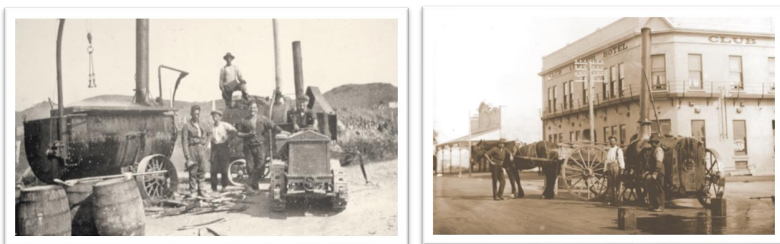
Horse drawn bitumen sprayer ready for sealing the main street of Opunake (right side photo)
