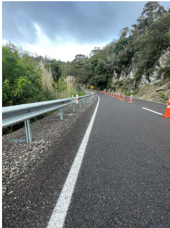
Mangamuka Road Guardrail Installation
