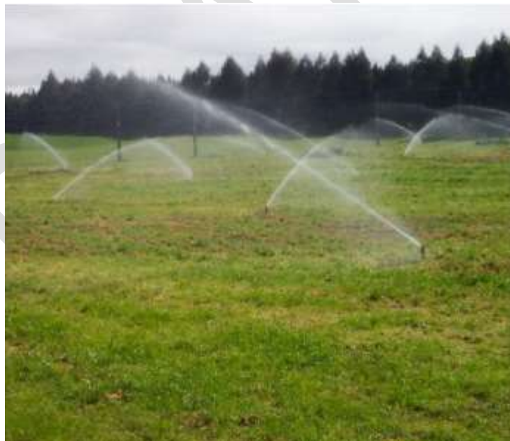
Figure 1211. Irrigation sprinklers operating at Taupo wastewater discharge site 17
