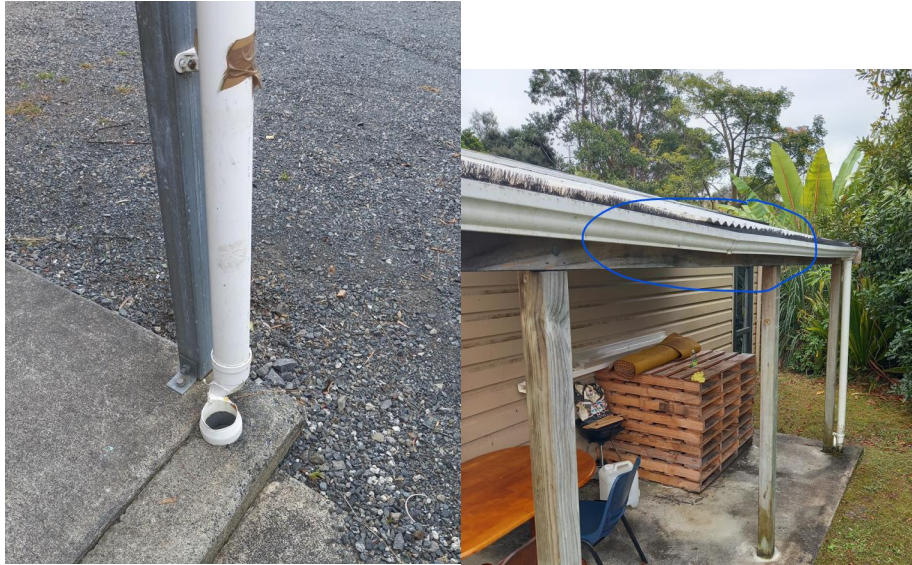
Down pipes/gutters were damaged in several areas. This can lead to erosion of footings and lead to subsidence if left uncorrected.
