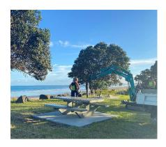
All our locations with new tables in Awanui, Kaitaia and Ahipara had Shade Systems come and install the poles for the star shaped umbrellas. The photos show the digger, drilling and preparing for concrete foundations to install the stainless steel pole shown below.
