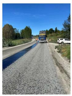
Figure 12: Oruru Rd Rehabilitation Site 2 Sealing
