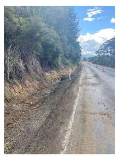
Figure 14: Kohukohu Rd Rehabilitation Water tabling
