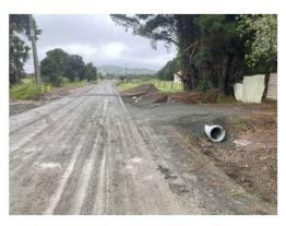
Figure 9: Parapara - Toatoa Rd Drainage Replacements
