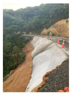
Figure 5: Peria Rd Seal Extension RP4100 Slip Repair
