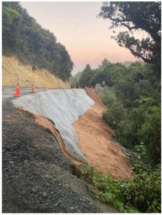
Figure 4: Peria Rd Seal Extension RP4100 Slip Repair
