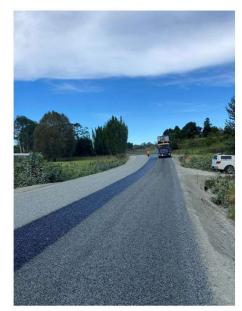
Figure 13: Oruru Rd Rehabilitation Site 2 Sealing
