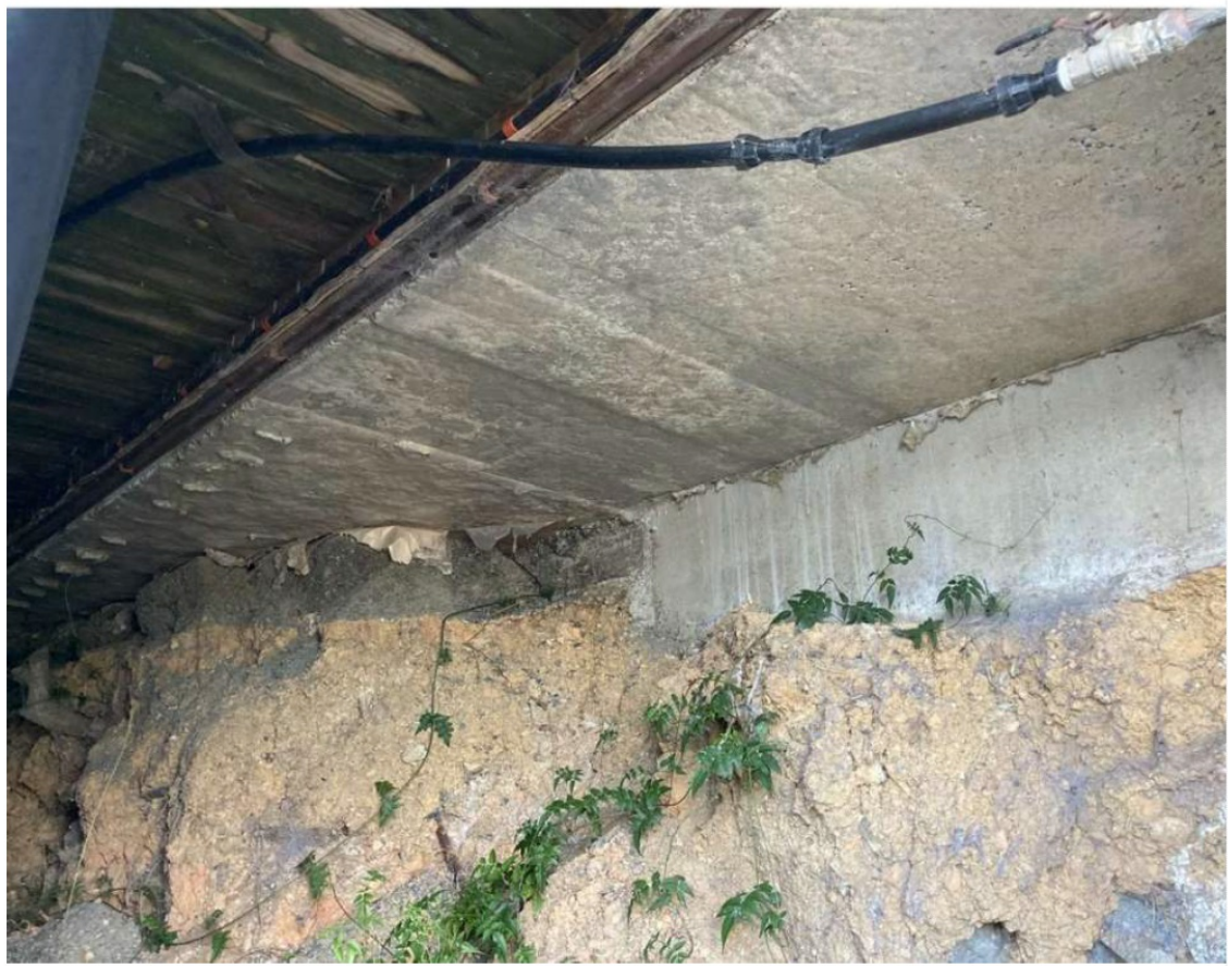
Photo 5: Close-out of the erosion of the soils undermining the foundation
