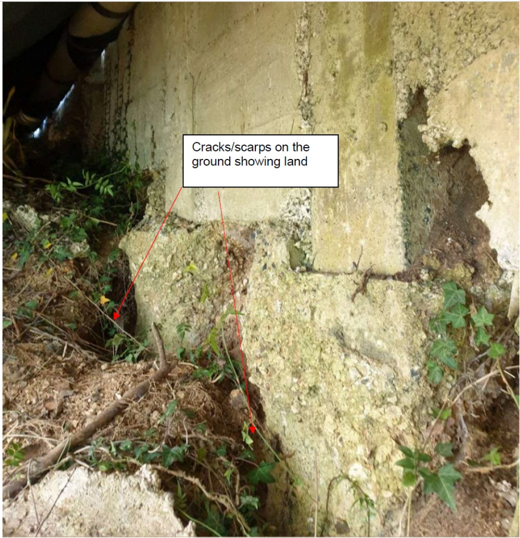
Photo 6: Close-out of the erosion of the soils undermining the foundation
