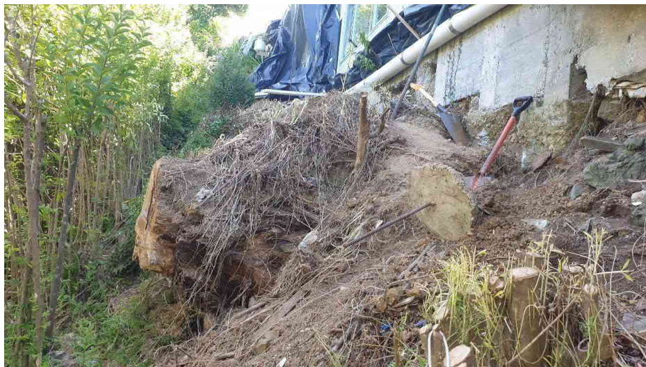
Photo 1: View to west along southern edge of dwelling showing exposed shallow foundation (right) and tree stump (left)
