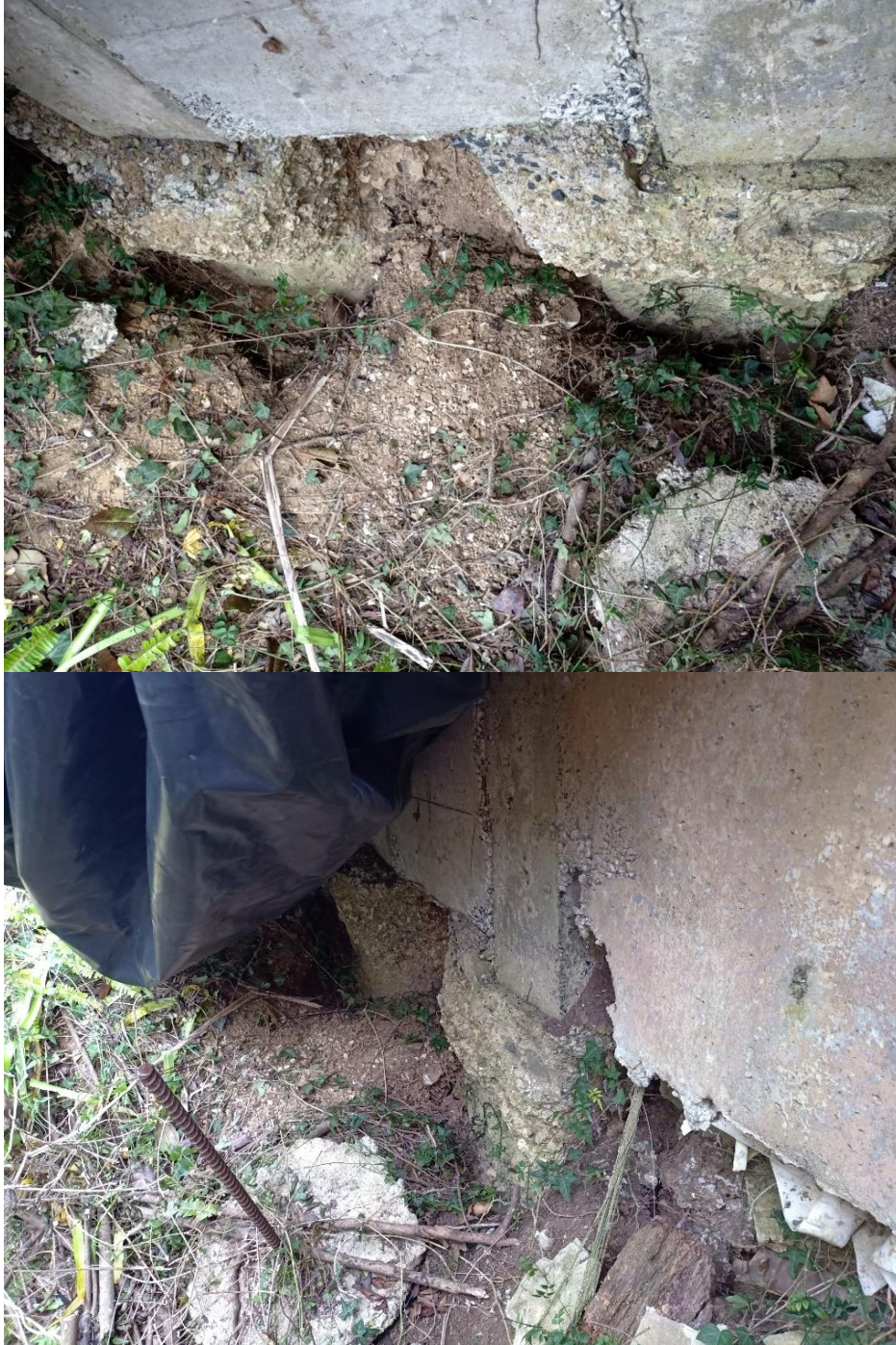
Photo 7: Exposed pile #2 & 3 showing scarp
