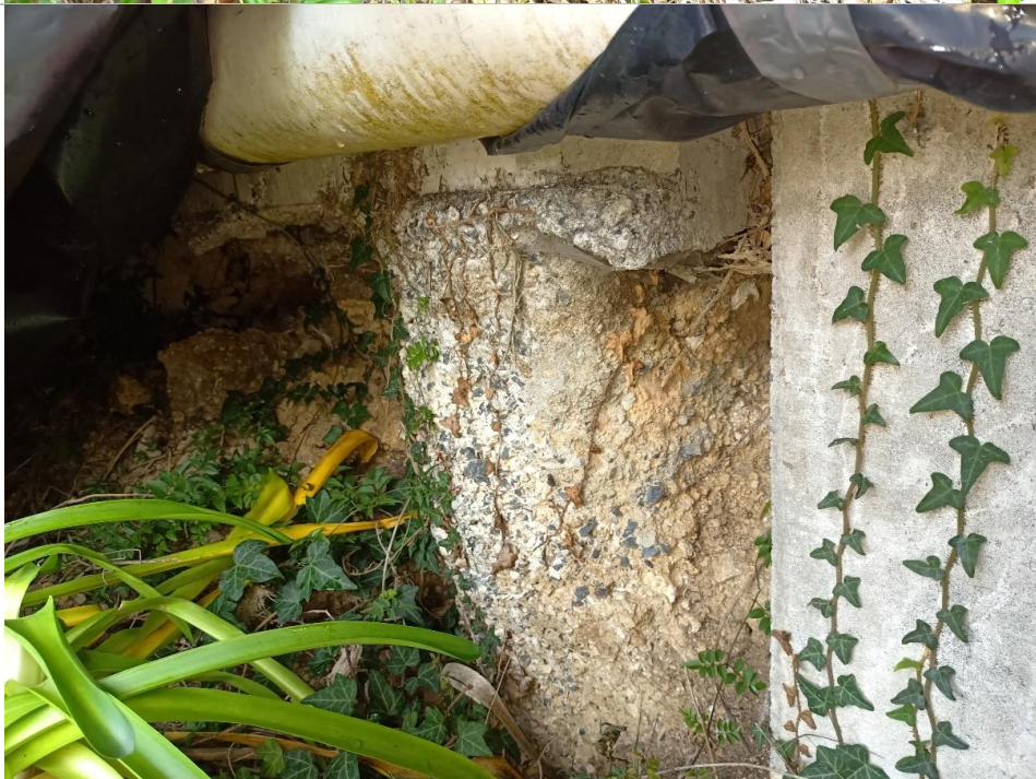
Photo 5: Western end where ground level is at concrete beam level Photo 6: Exposed pile #1
