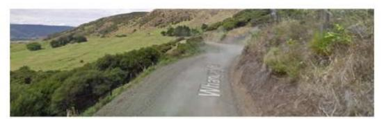
Figure 35: Whangape Road narrow winding / tortuous unsealed section.
