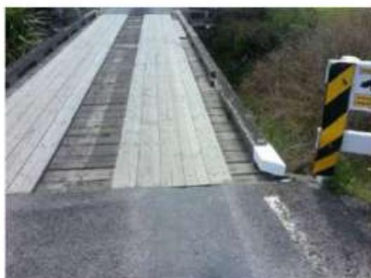
*Quarry Rd, Kaikohe – Bridge Repairs to edging and running boards*
