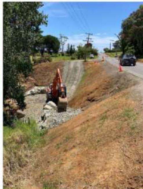
Figure 8: Oruru Rd Rehab & Rockwall In Progress
