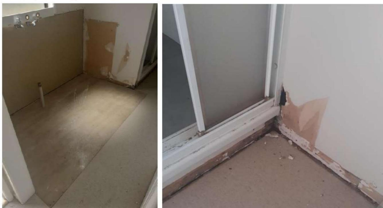
*Unit 2, Waima washtub removed, damaged wall lining, and flooring replaced*
