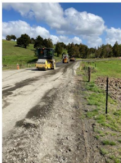
Figure 12: Pawarenga Rd Rehab Stabilising
