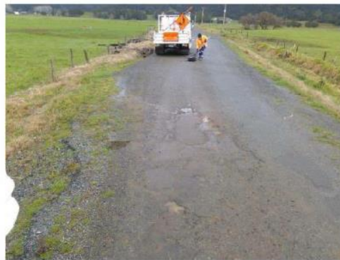
Hariru Rd – Pothole repairs being carried out by Marie & Kahu
