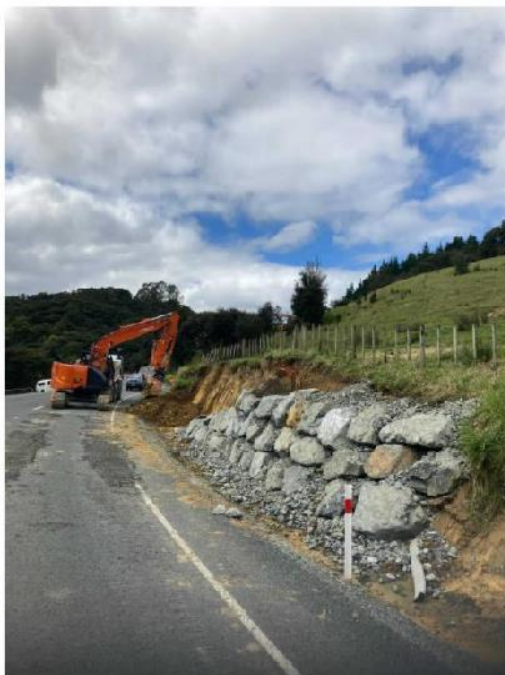
Figure 5: Peria Rd Seal Extension Slip Repairs
