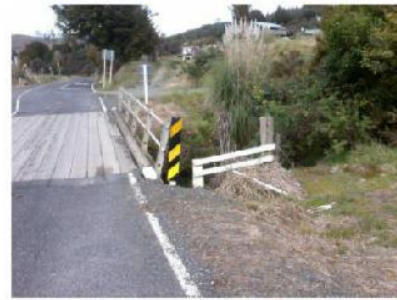
Pipiwai Rd – Missing Bridge End Marker Installed
