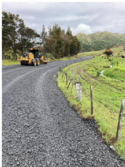
Figure 10: Pawarenga Rd Rehab Pavement Overlay
