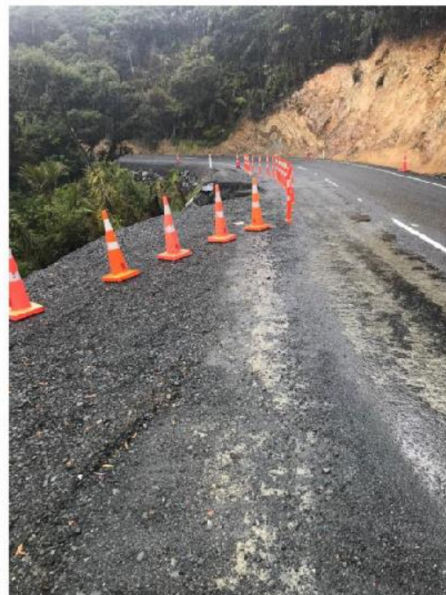
Figure 8: Peria Rd Underslip delineation
