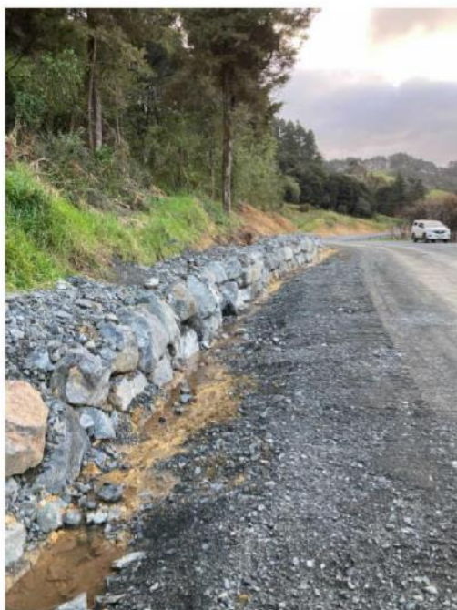
Figure 7: Peria Rd Seal Extension Toe Support
