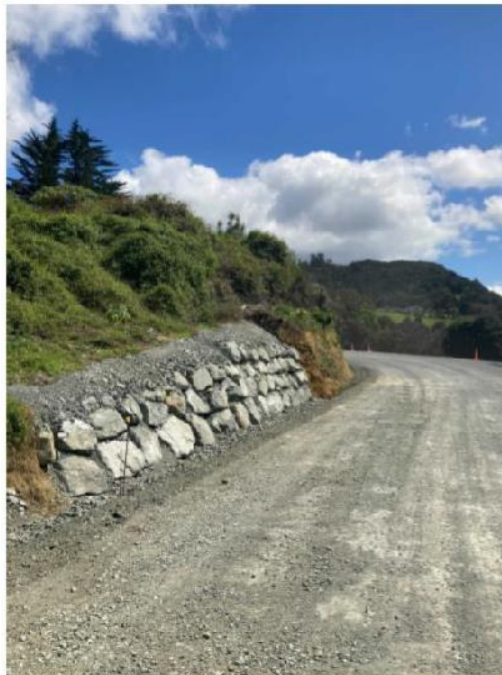
Figure 6: Peria Road Seal Extension Slip Repairs
