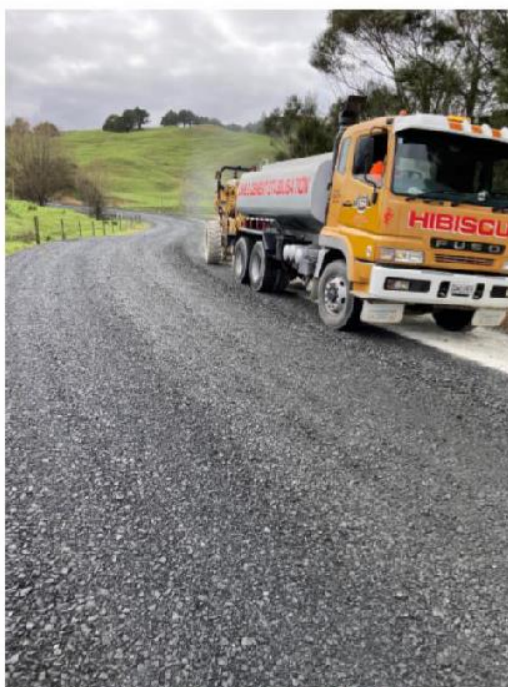
Figure 14: Pawarenga Rd Rehab Stabilising
