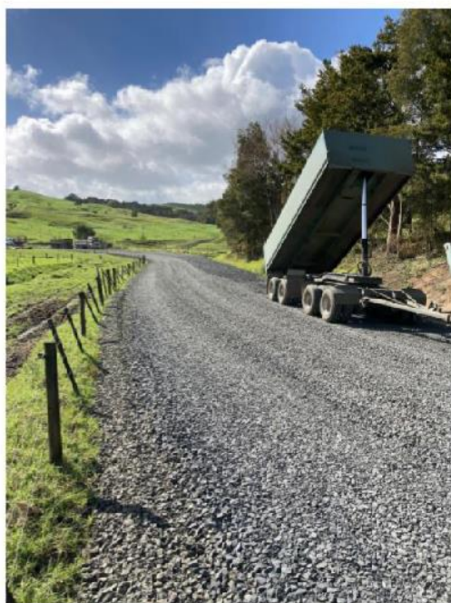
Figure 11: Pawarenga Rd Rehab Pavement Overlay
