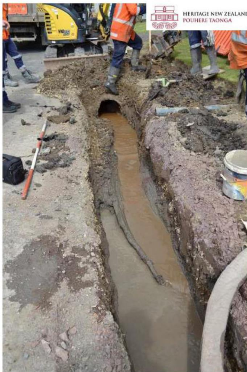
Figure 6: Once the Ventia team opened up the blocked concrete pipe culvert, the water flowed out and through the wooden item. This suggested that the item was part of a rotted tree laid in the swale drain that would have run alongside the old road and assisted in the transportation of water away from the adjacent properties. The lack of any construction adzing and the 'kink' in the item (visible here) confirms that that this was not built and would not function as a waka. It does however function as a culvert as is clearly visible here.
