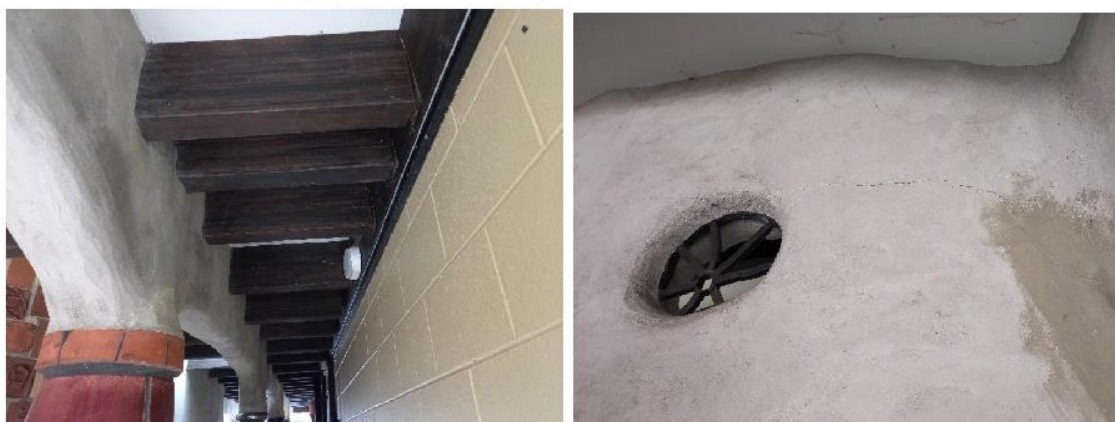
Hundertwasser Toilets with cracking in plaster work and wooden beams pulling away from neighbouring building
