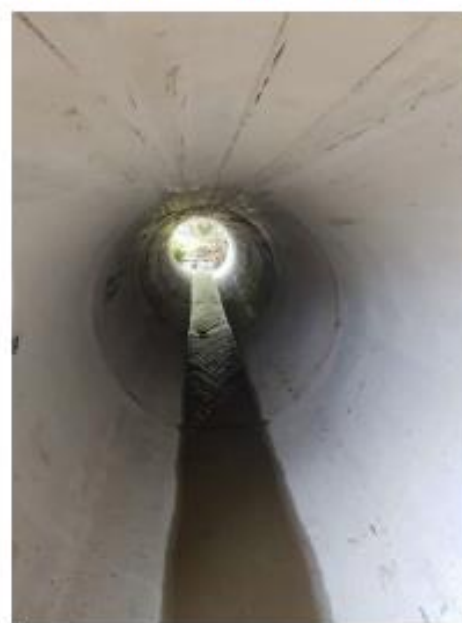
Wallis Rd – Large diameter Culvert installed
