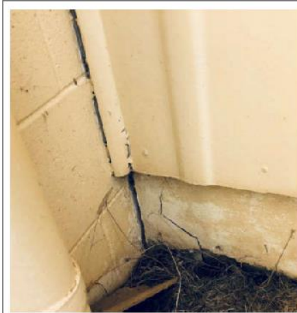
Crack in foundation between units A and B. All the crack patterns are similar and indicating the development of stresses in the structure due to differential settlement.
