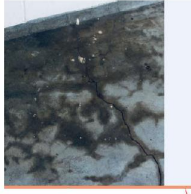
Cracks in front concrete slab (Unit B)
