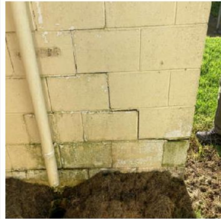
Cracks in the concrete wing wall at rear side of unit A. The wing wall is partly supporting the roof system. (Settlement due to shrink swell of soils) – north-eastern wall
