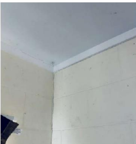
A similar crack show above extended inside the structure.
