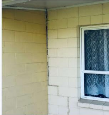
Cracks in concrete front wall (Unit B, A & B) due to differential settlement. The cracks are extending from top to bottom and progressing further into the foundation. Refer to the photo on the right for the development of cracks in the slab.
