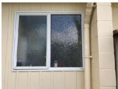
Windows are racked due to settlement of building
