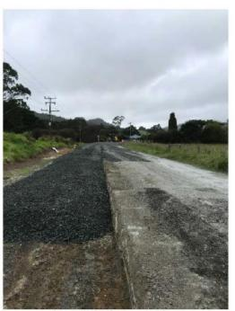
Figure 7: Section Five Pavement undercut
