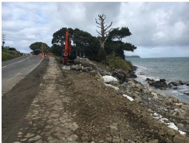
Photograph 2.4c: NZTA seawall currently under construction
