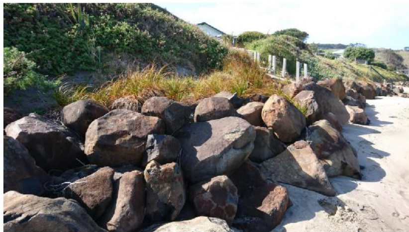
Photograph 2.4a: Riprap armouring north of site
