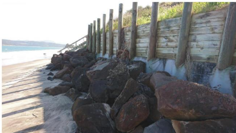
Photograph 2.4b: Combination rock rip-rap and timber armouring
