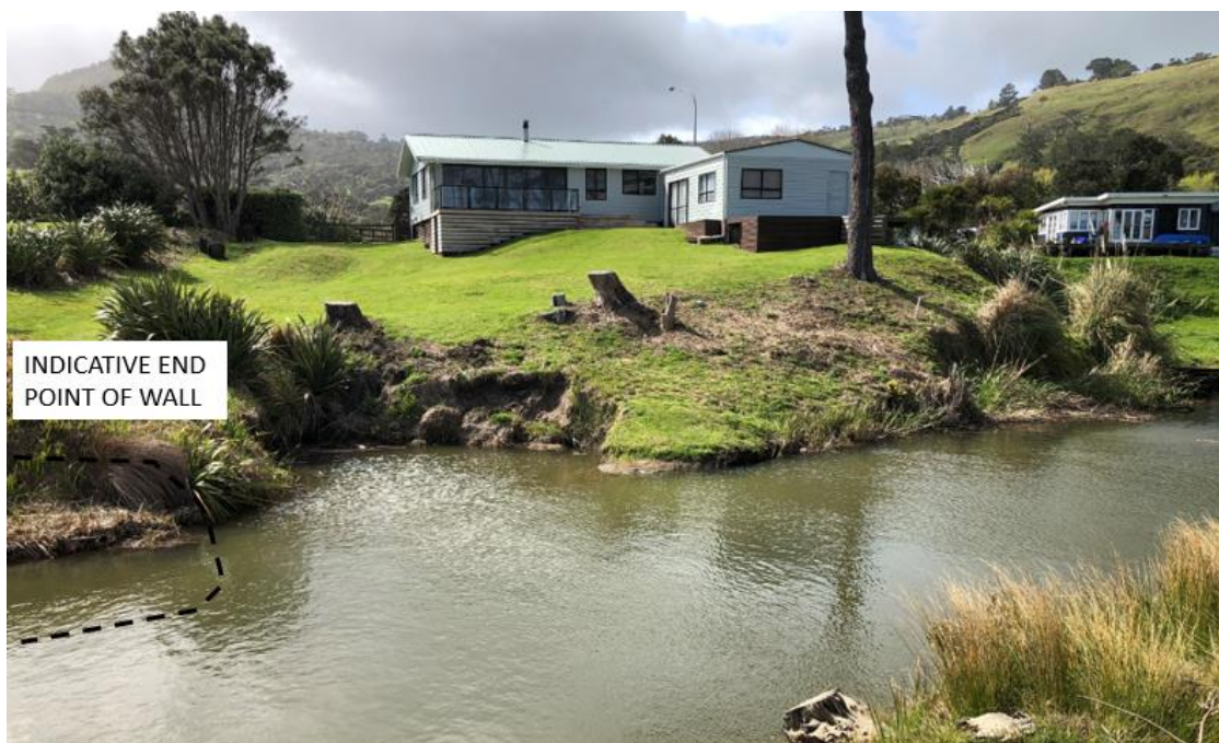
Photograph 8.6.2a: Indicative upstream end to wall
