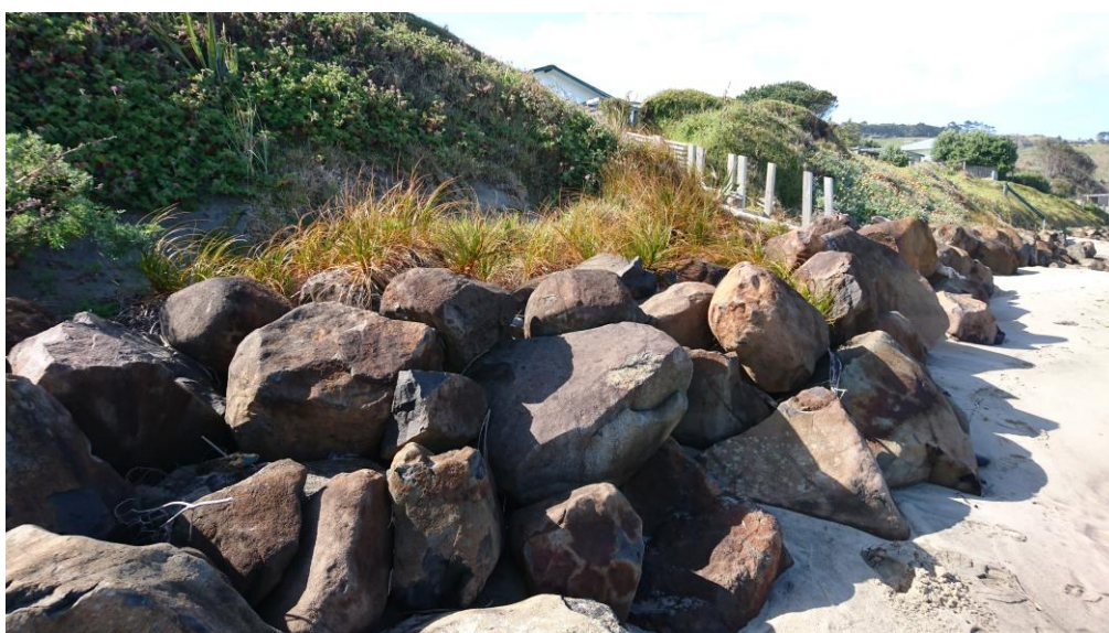
Photograph 2.4a: Riprap armouring north of site
