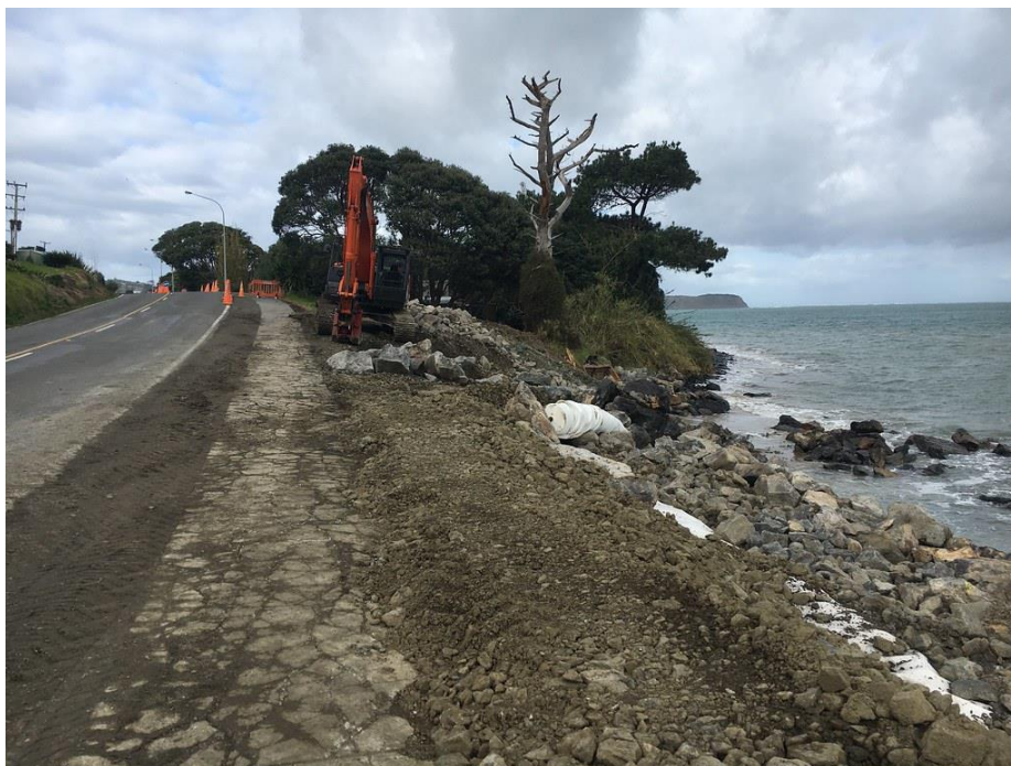
Photograph 2.4c: NZTA seawall currently under construction
