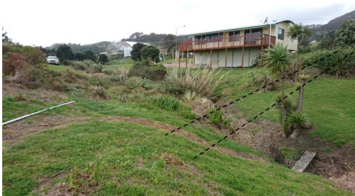
Photograph 8.4: Indicative location of public access to Reserve
