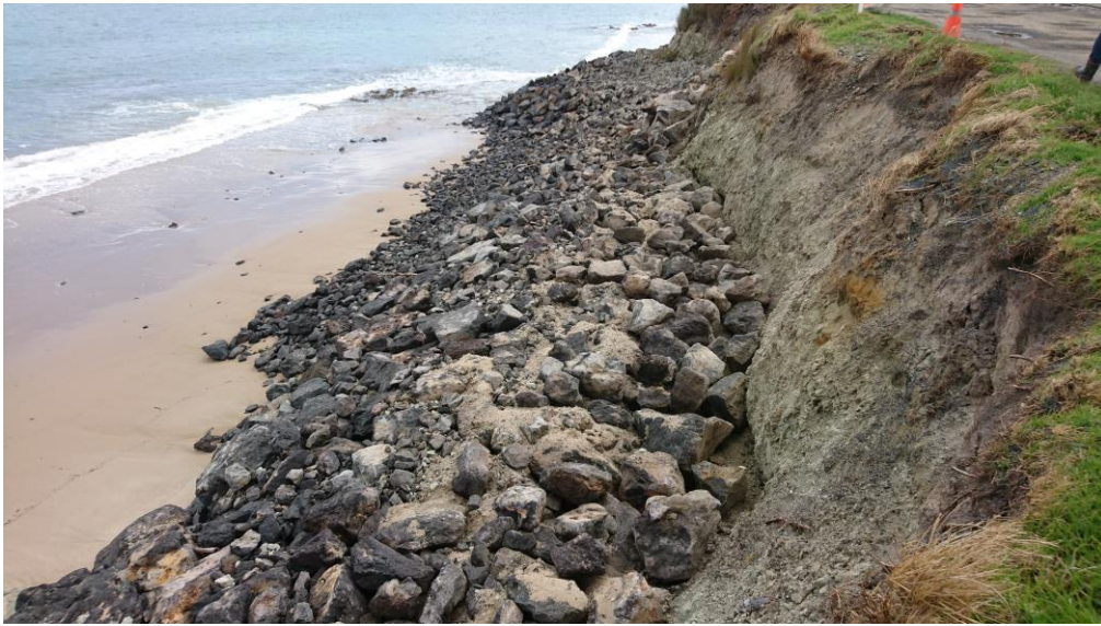
Photograph 2.4d: Small rock present in face of new NZTA seawall
