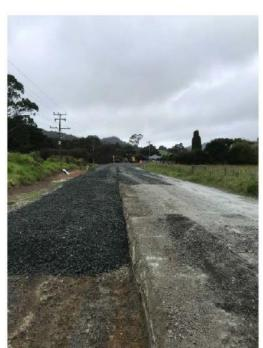
Figure 7: Section Five Pavement undercut
