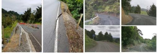
A key challenge to the network is resilience – slumps and dropouts are prevalent. An associated concern is the inconsistent and damaged safety/warning devices used to keep road users safe.
