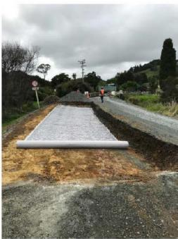
Figure 6: Section Five Bridge Undercut
