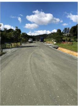
Figure 22: Section Four Drag Brooming
