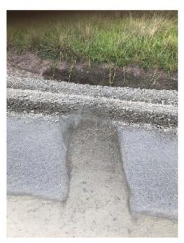
Figure 4: Great compaction all the way to edge of shoulde
