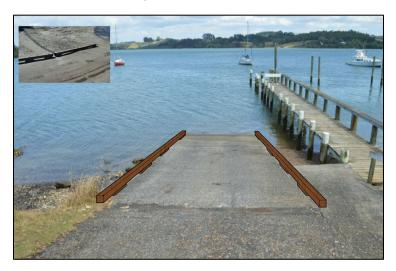
The Rangitane Wharf structure is not safe for docking boats and boats approaching the ramp have to come aground on the concrete ramp.
