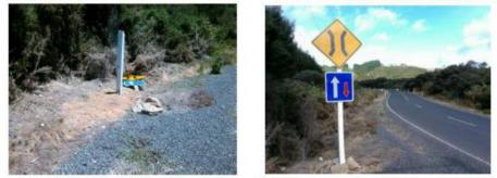
Kerikeri Inlet Rd - Vandalism - Before and after. Note post has been cut with a saw.
