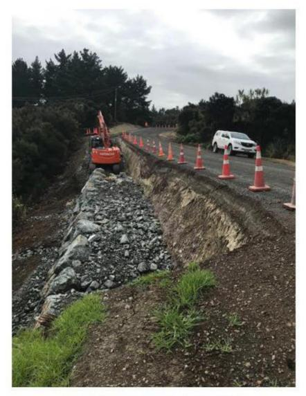
Figure 1: Rock wall construction in progress
