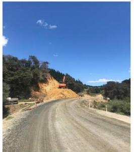
Figure 4: Clearing and corner widening in Section Four
