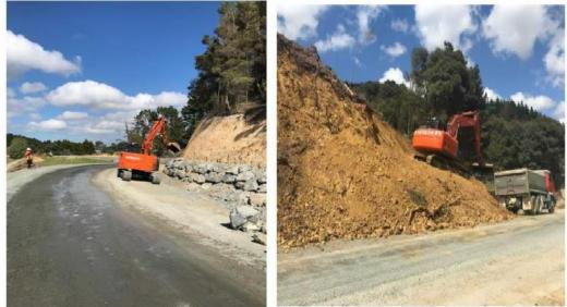
Figure 2: Construction of rock wall in Section 3.
