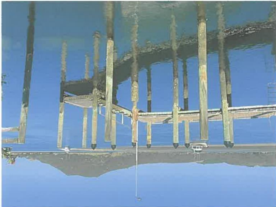
Wooden wharf at low tide showing wet loading platform stairway and wooden piles. Club volunteers have attempted to strengthen rotten pile by pouring concrete around it.
