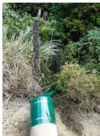
Cabbage Tree Bay Rd – Culvert sock installed on end of pipe extension following storm event
