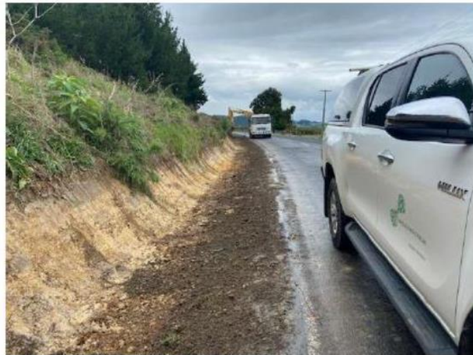
Horeke Rd – Water tabling.
