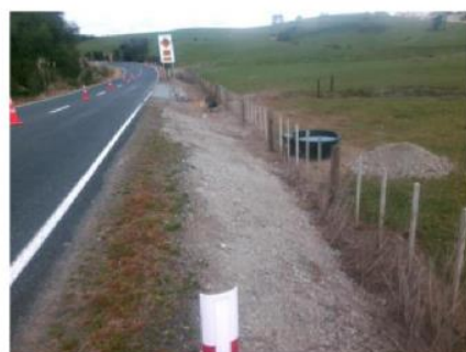
Ngunguru Rd Concrete shoulder repairs
