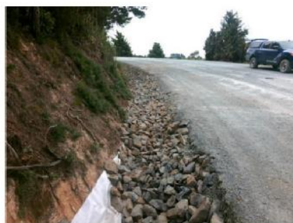
Mine Rd Stage 1 Water table reconstruction
