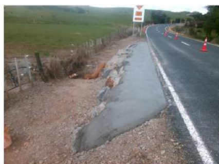
Ngunguru Rd Concrete shoulder repairs
