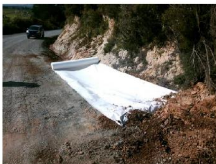
Mine Rd Stage 1 Water table reconstruction
