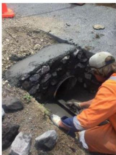
Lance installing a headwall on Blacks Rd
