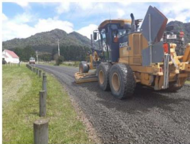
Waima School Rd dust seal – stabilising and chipseal to follow in early Nov
