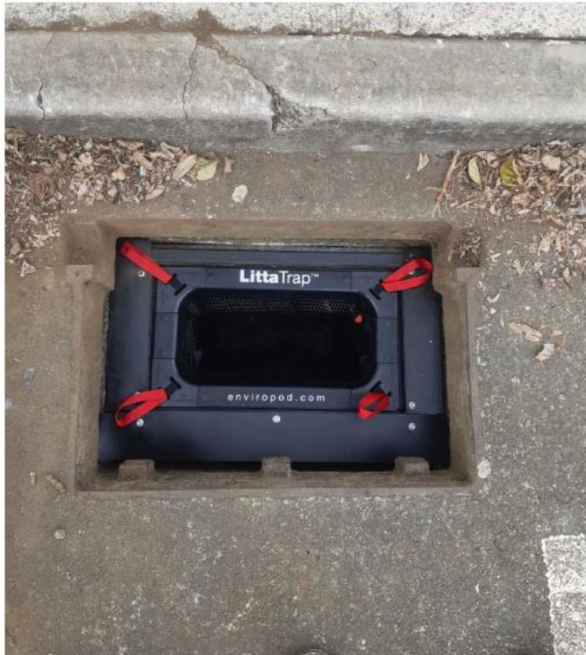
Enviropod Litta Trap installed in cesspit on behalf of NRC/Northtec
