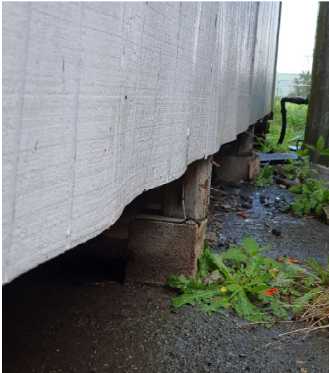
Figure 16 Deformed shadowclad ply cladding
