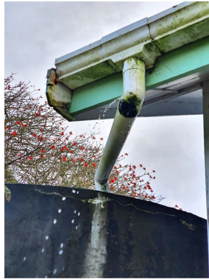
Figure 23 Gutter showing leak
