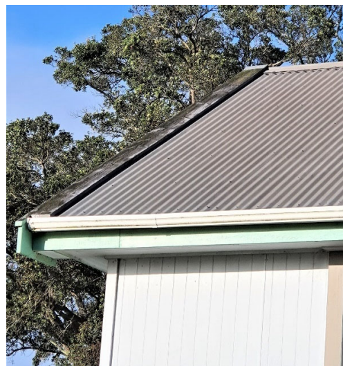
Figure 21 Roof showing algae build up
