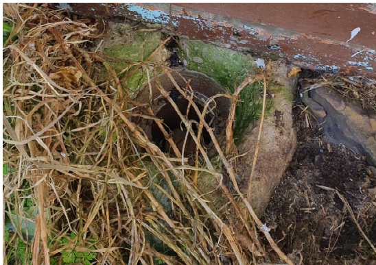
Figure 48 Kitchen gully trap overgrown
