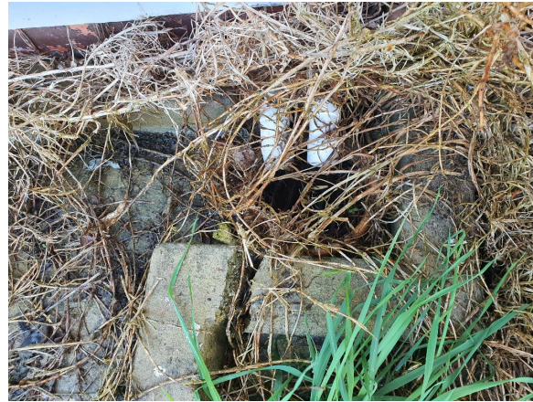
Figure 47 Toilet gully trap overgrown & damaged
