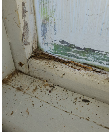
Figure 29 Rotten interior windows
