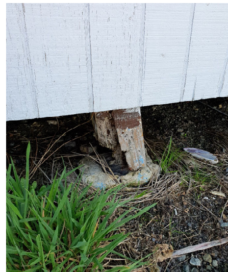
Figure 9 Rotten perimeter foundation pile
