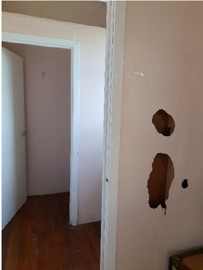
Figure 28 Damaged wall linings
