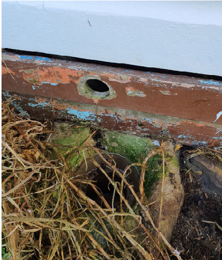
Figure 40 Sink waste not connected to outside
