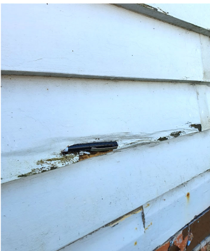
Figure 14 Rotten weather boards
