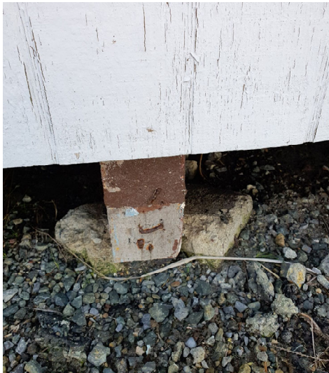
Figure 8 Degraded perimeter pile footing
