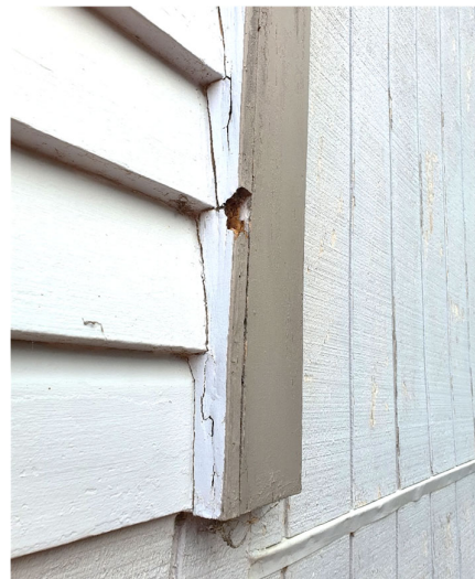
Figure 15 Rotten mouldings
