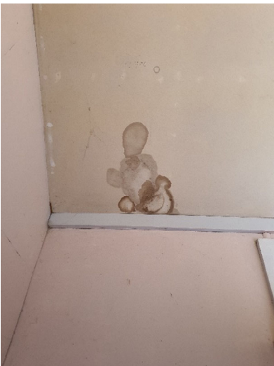
Figure 26 moisture on ceiling lining
