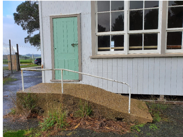
Figure 41 Non-complying ramp to building
