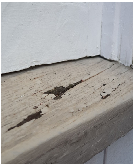
Figure 18 Typical rotten window sill
