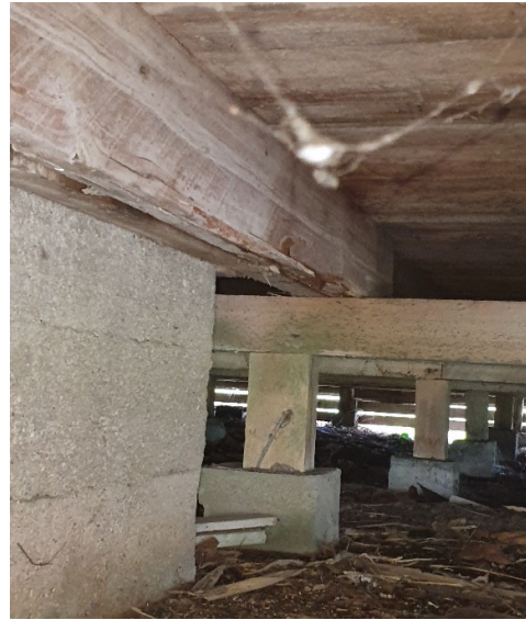
Figure 11 Pile footings and subfloor framing 2
