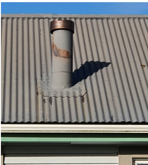
Figure 20 Roof showing disused flue
