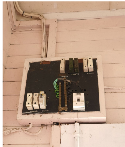
Figure 37 Electrical subpanel
