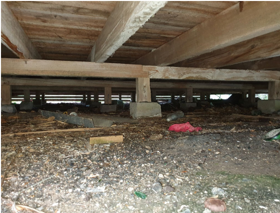
Figure 10 Pile footings & subfloor framing 1
