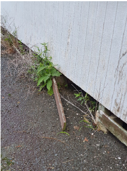
Figure 12 Damaged baseboards
