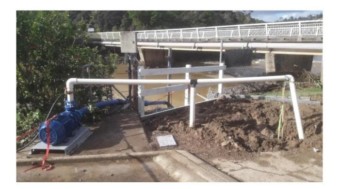
The water level during this event reached 200mm up the side of the water treatment plant building at the height of the flood. The plant remains on temporary supply with subsequent weather events and water conditions making conditions unacceptable for diving operations to affect repair.
