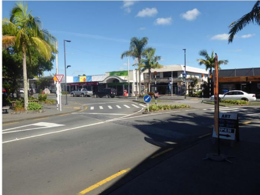
Figure 5 : Pedestrian Crossings on raised platforms at the intersection of Cobham Road and Kerikeri Road.
