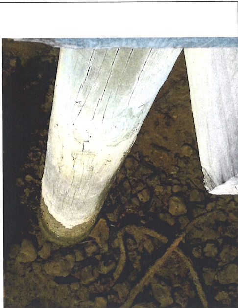
Figure 13 Pile for 880 mm boardwalk section
