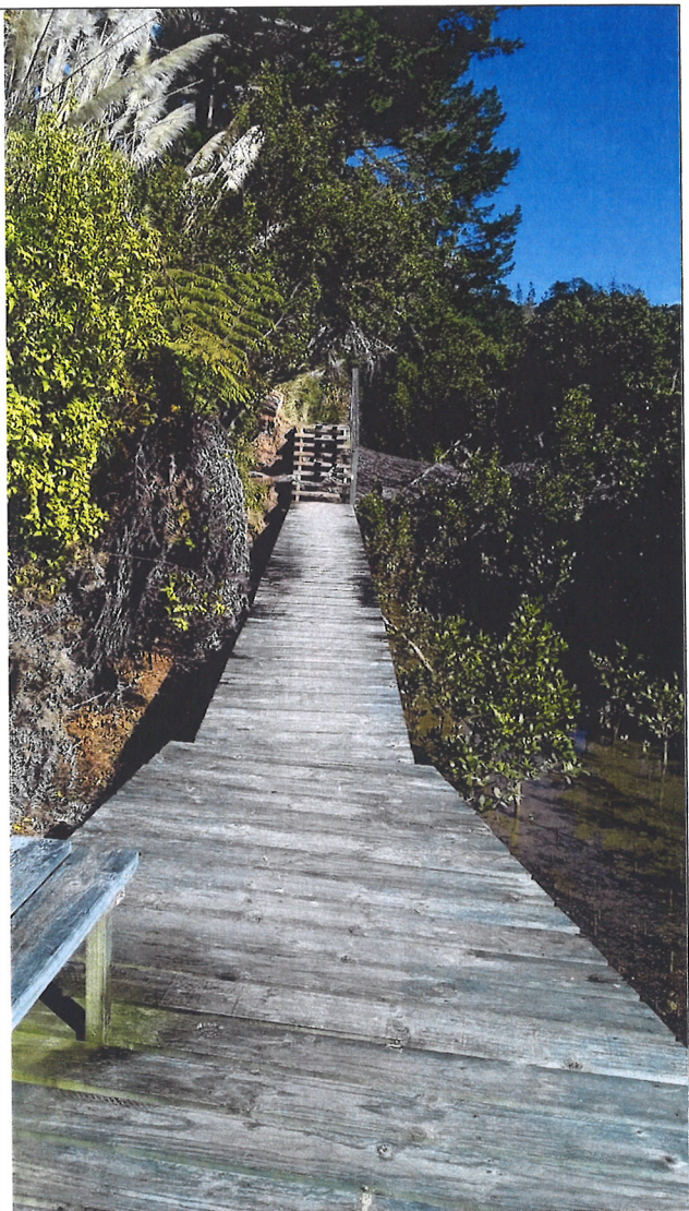
Figure 14 880 mm Boardwalk section
